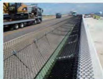
橋梁落下物防止網
